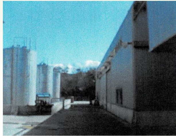
Inside View of the plant
