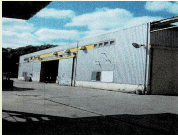
Outside of the plant
