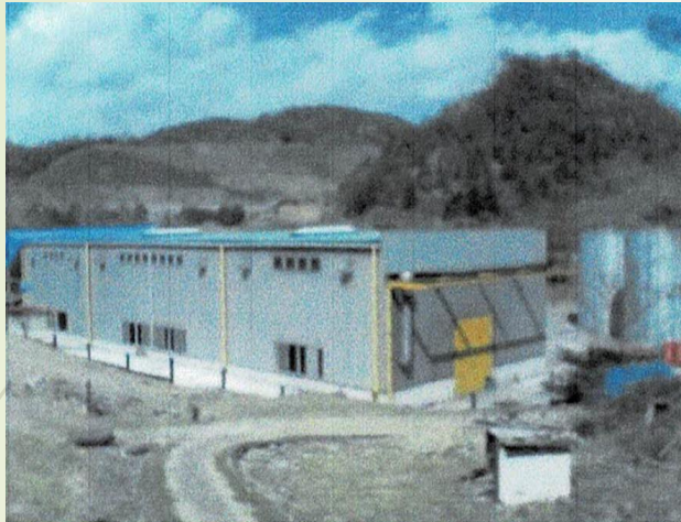
Overall view of the plant
